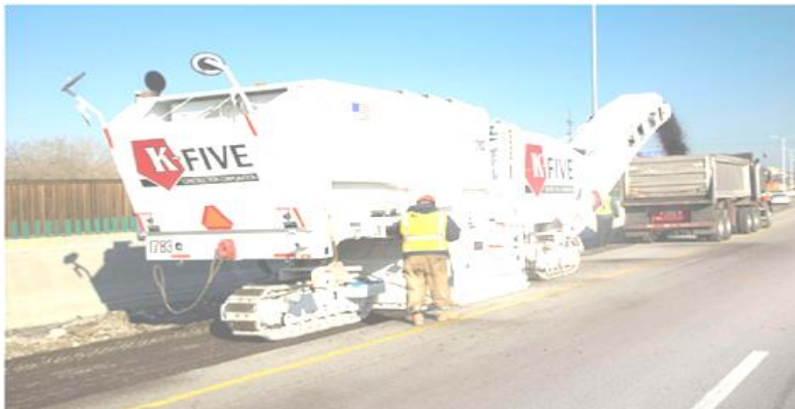
Figure 2.1: Site process of reusing binder course (Randy, 2010)
